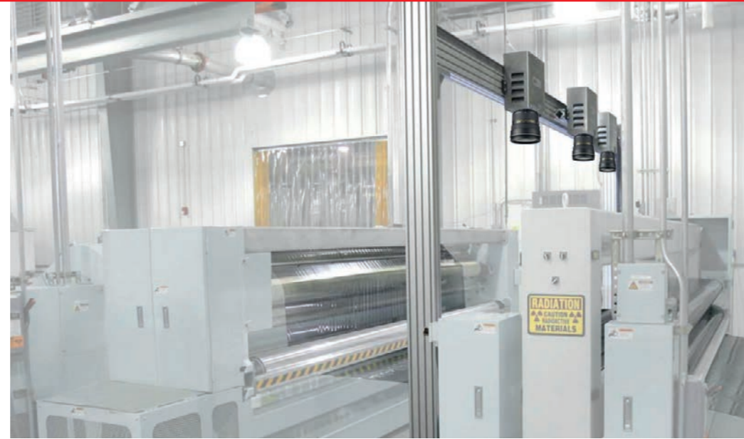
PET film extrusion with optical quality control system (source: OCS GmbH)
